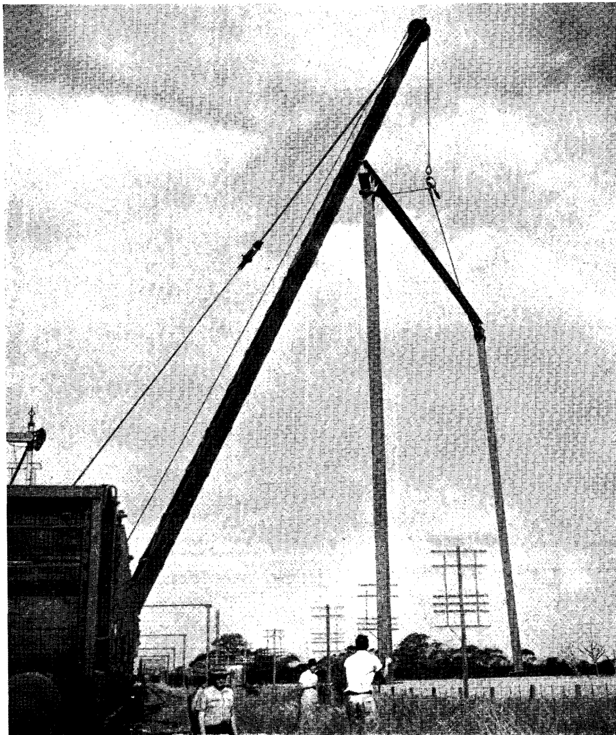
Erecting Overhead Structures on the Gippsland Line.
